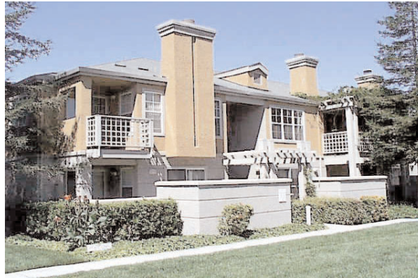
Individual residences are articulated through the use of variation in the massing, recessed balconies, wall breaks and varying roof forms.
