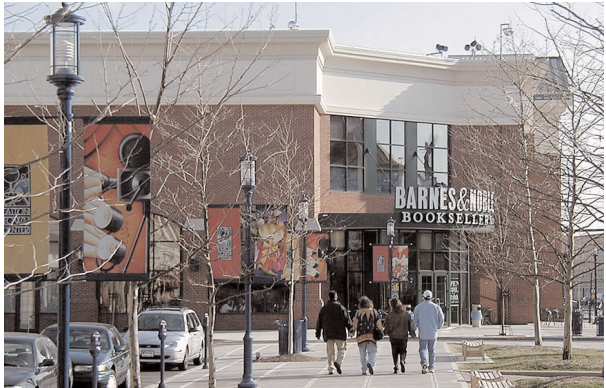
A distinctive cornice enhances the roof line.
