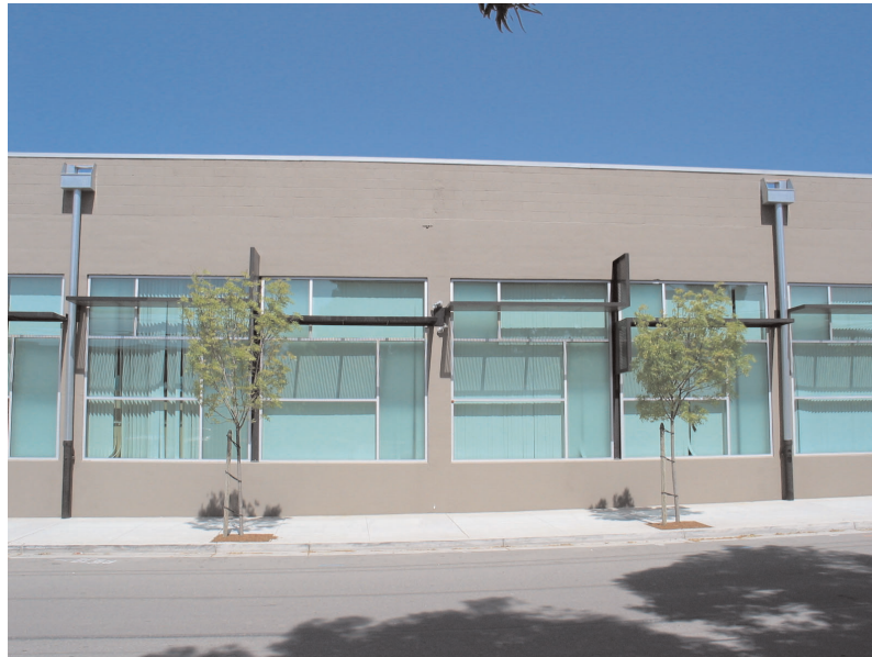
Sun screens reduce the amount of direct sunlight that enters a building.
