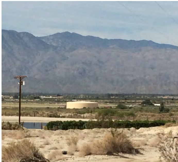
Figure 3-7: View of One of the Above-ground Water Tanks in the Coachella General Plan Area
