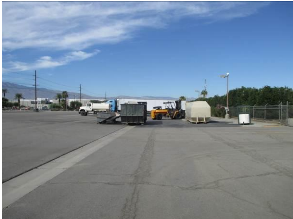
Photo #7 Additional view the asphalt-paved area looking west.
