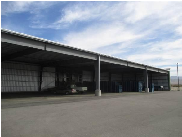
Photo #13 View of storage shed located on the northeastern portion of the northern parcel looking northeast.
