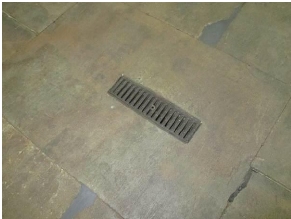
Photo #27 Typical view of interior floor drain in the warehouse area.
