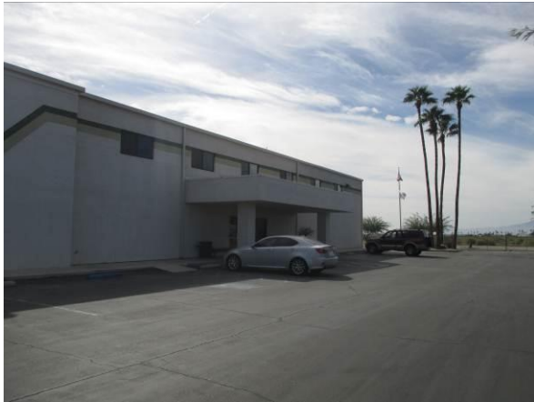
Photo #19 Exterior view of the Valley Pride office space on the southwestern portion of the building.
