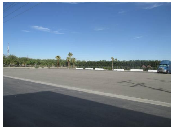
Photo #6 View of asphalt-paved parking area on the northern portion of the northern parcel.
