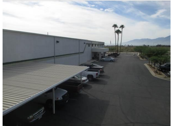
Photo #14 Typical view along the southwestern portion of the northern parcel looking south.
