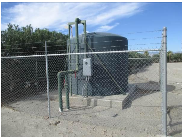
Photo #47 View of the 5,000-gallon water AST used for storage of waste water generated on the site, and then sprayed on the vacant land.
