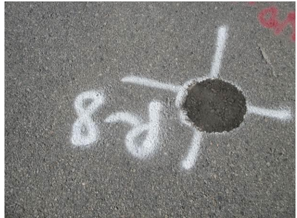
Photo #50 Typical view of asphalt-patched soil boring observed during the site reconnaissance.
