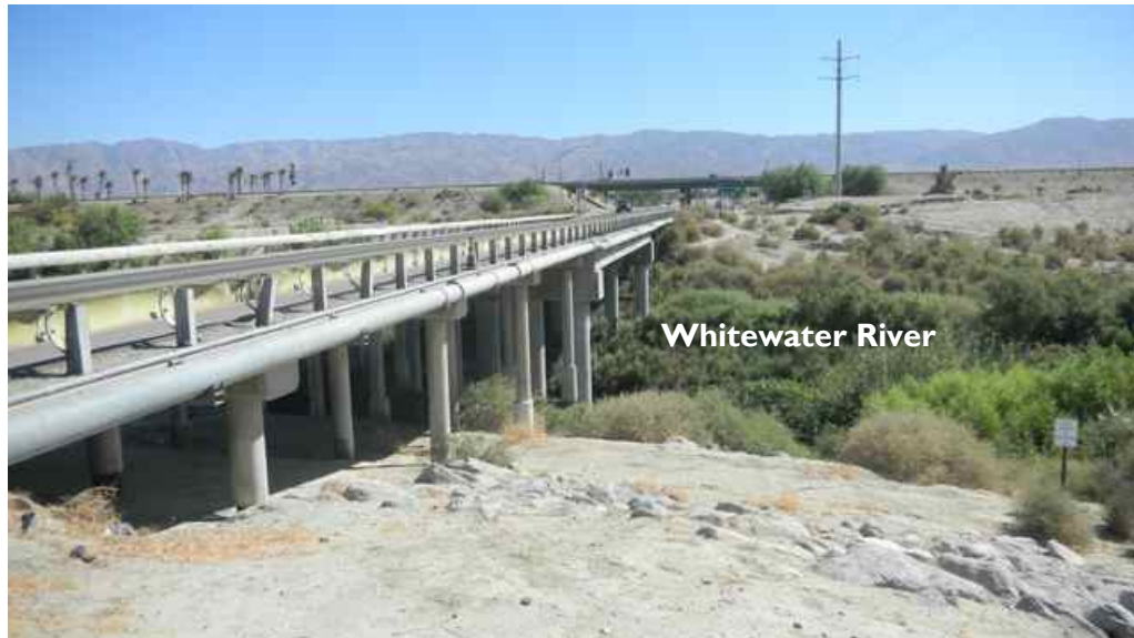
Figure 3-4: Bridge Crossing the Coachella Valley Stormwater Channel (Whitewater River) at Dillon Road
