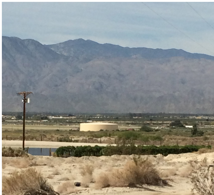
Figure 3-7: View of One of the Above-ground Water Tanks in the Coachella General Plan Area
