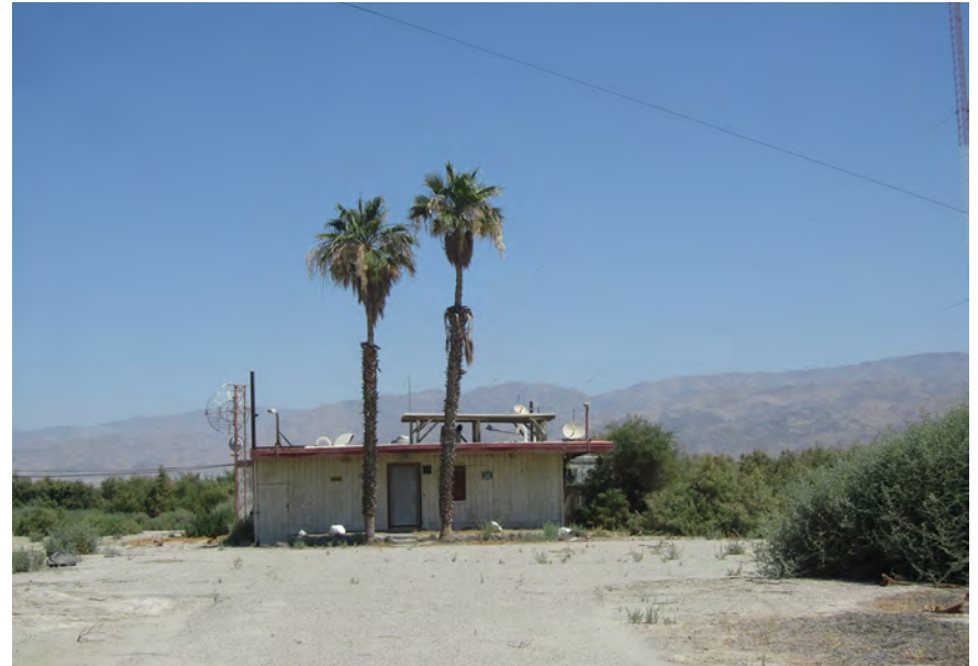
View of an existing radio tower station located along 50th Avenue to the east of SR-86.
