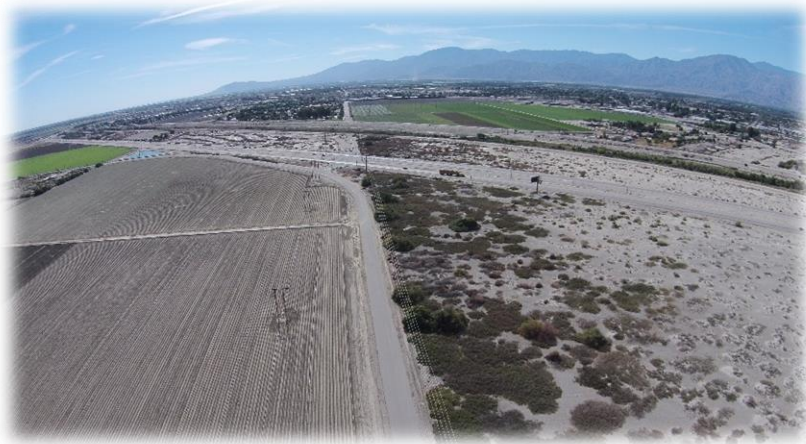
Western view of the project at the SR-86/Avenue 50 Interchange
