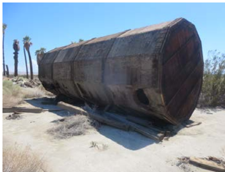
WOODEN AST NEAR THE NORTH PROPERTY BORDER, LOOKING SOUTHEAST
