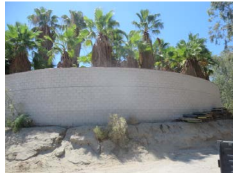
WEST ADJACENT CORONA YACHT CLUB, LOOKING WEST FROM THE PROPERTY
