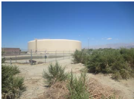
WEST ADJACENT WATER TOWER, LOOKING NW FROM THE SW PROPERTY CORNER
