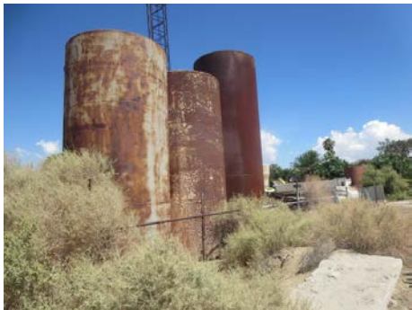
EMPTY ASTS ON THE NORTH ADJACENT SCRAP METAL YARD, LOOKING NORTHEAST
