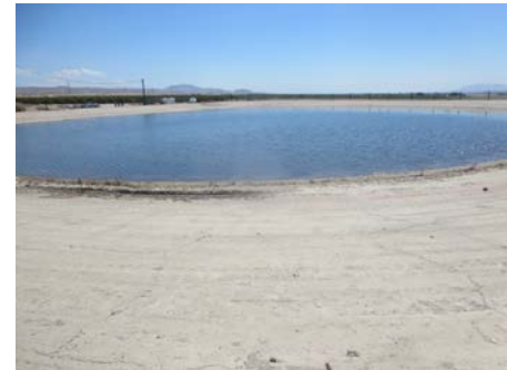
WATER RETENTION POND ALONG THE NORTH PROPERTY BORDER, LOOKING NORTHEAST
