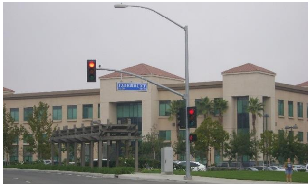
Typical two-story office building.
