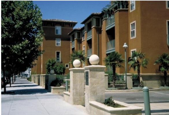
Three-story apartment complex with a landscaped setback.
