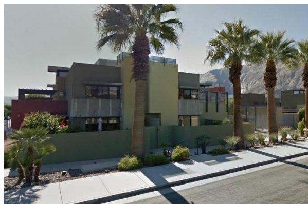
Three-story modern townhouses with tuck-under parking.
