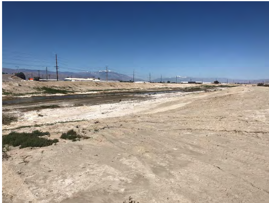
Coachella Valley Stormwater Channel, facing northwest, March 30, 2020
