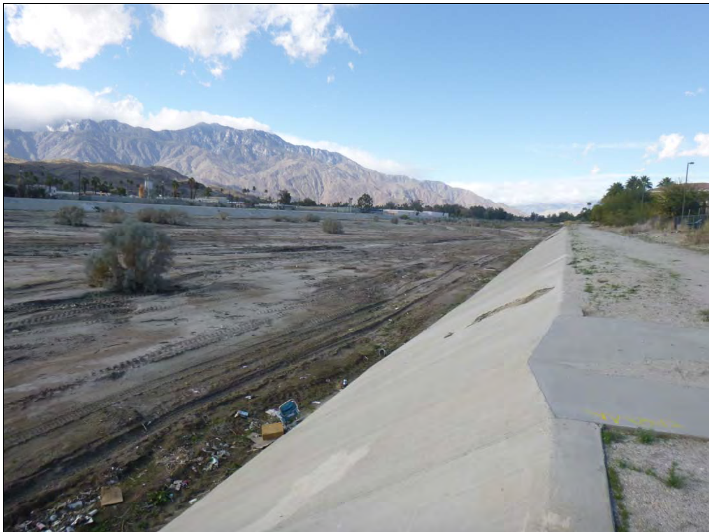
Channelized segment of the CVSC with cement-lined slopes between Frank Sinatra Drive and Cathedral Canyon Drive (view to the northwest; photograph taken January 10, 2017).
