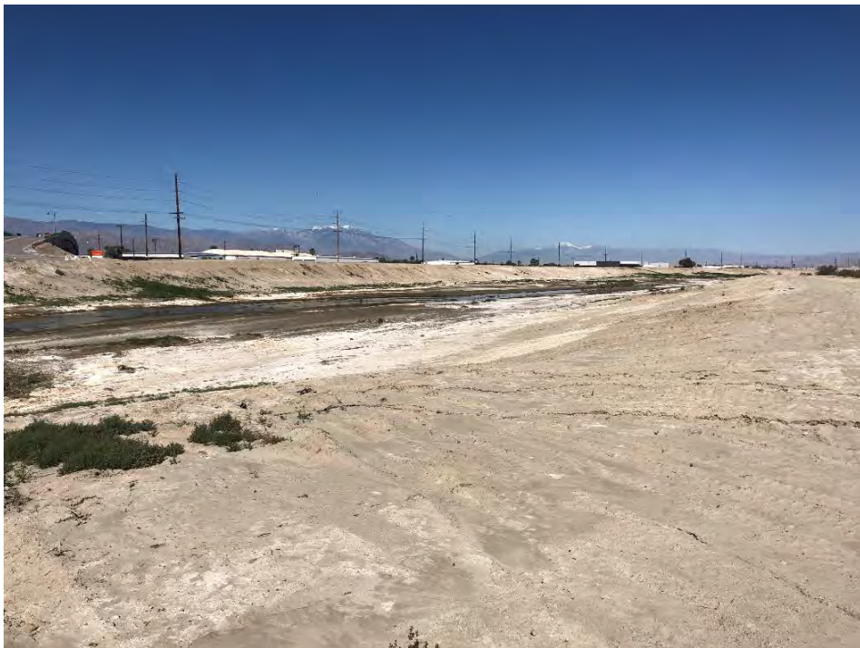
Figure 5-4 Overview of the stormwater channel from the survey area, view to the northwest
