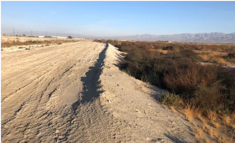
Photograph 8. Facing north, showing the start of the berm on the west side of the site that separates the site from the Whitewater River/ Coachella Valley Stormwater Channel
