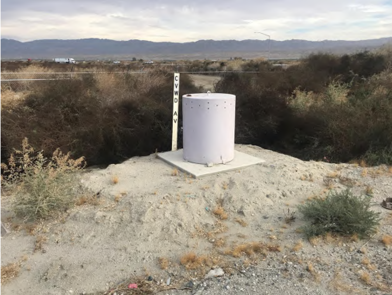
CVWD water well located along the Whitewater River channel, west of the TP, along Airport Blvd.
