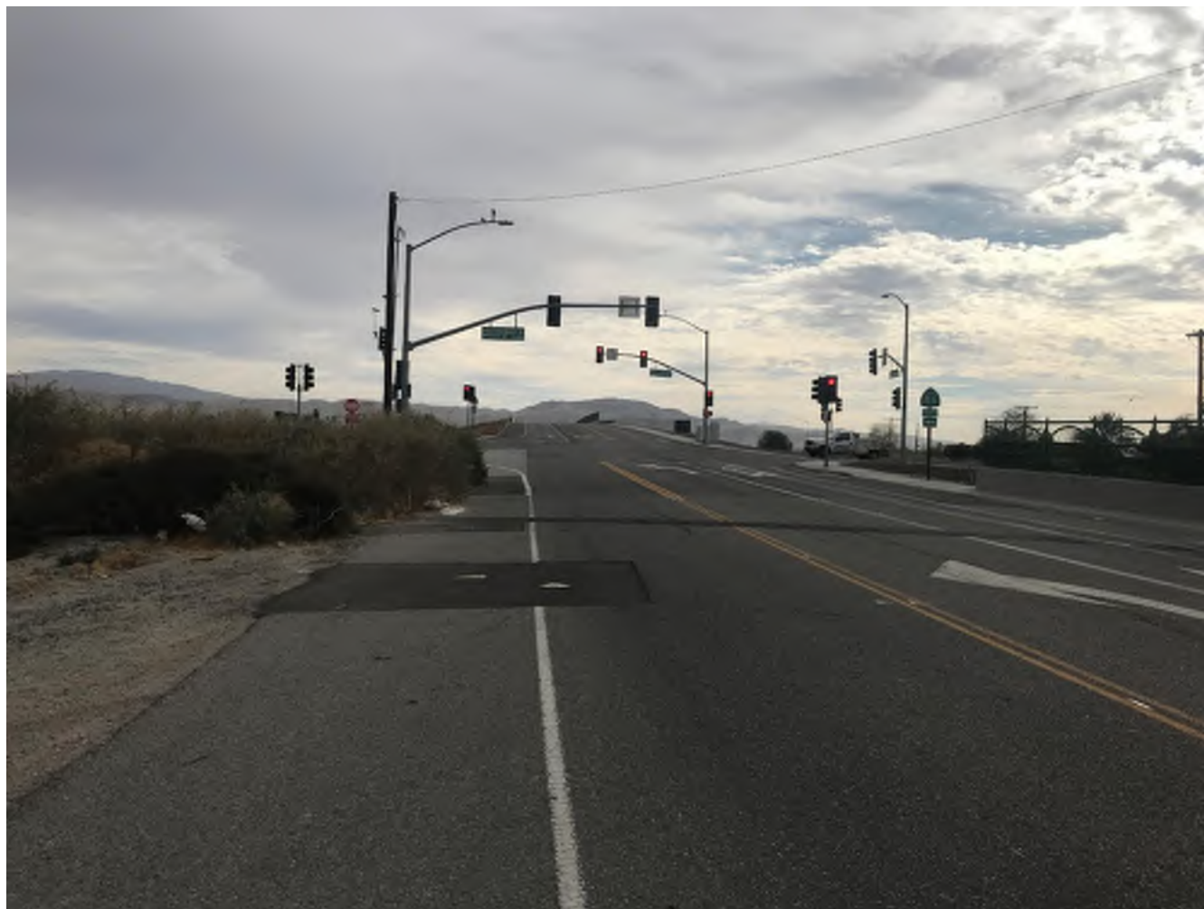
View to the east along Airport Road (south edge of TP) towards Highway 86.
