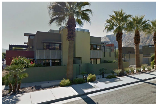
Three-story modern townhouses with tuck-under parking.
