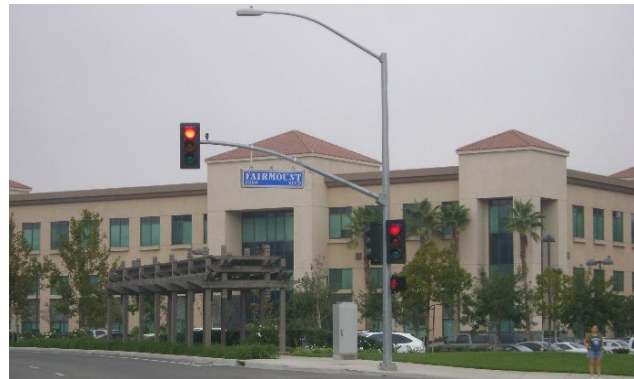
Typical two-story office building.
