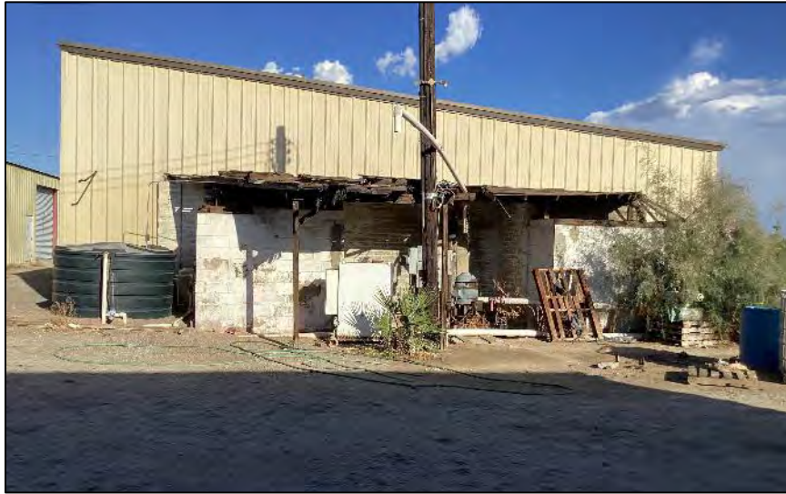
Photograph 23: West elevation of Building E. Camera facing east, October 6, 2022.
