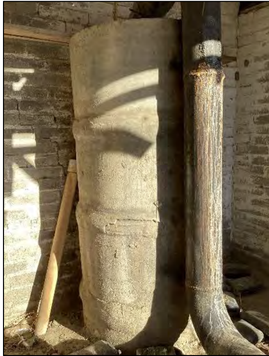
Photograph 4: Concrete cistern located behind the inactive irrigation pump. Camera facing southeast, October 6, 2022.
