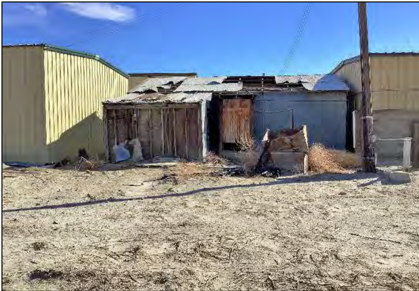
Photograph 20: North elevation of Building D. Camera facing south, October 6, 2022.
