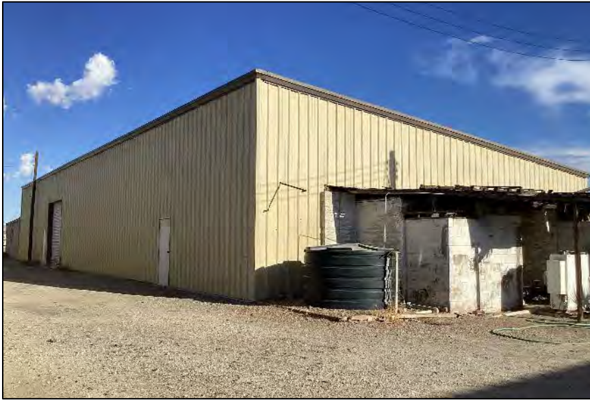
Photograph 29: North side and west end of Building J. Building E is at the far right side of the frame. Camera facing southeast, October 6, 2022.
