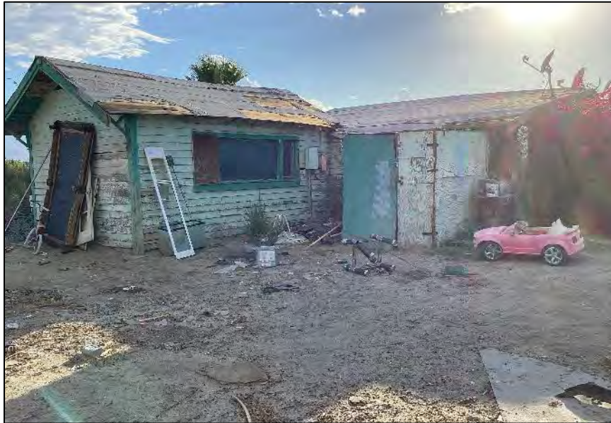
Photograph 12: North side of the gabled addition (left) and the modern plywood enclosure (right). Camera facing southwest, October 6, 2022.
