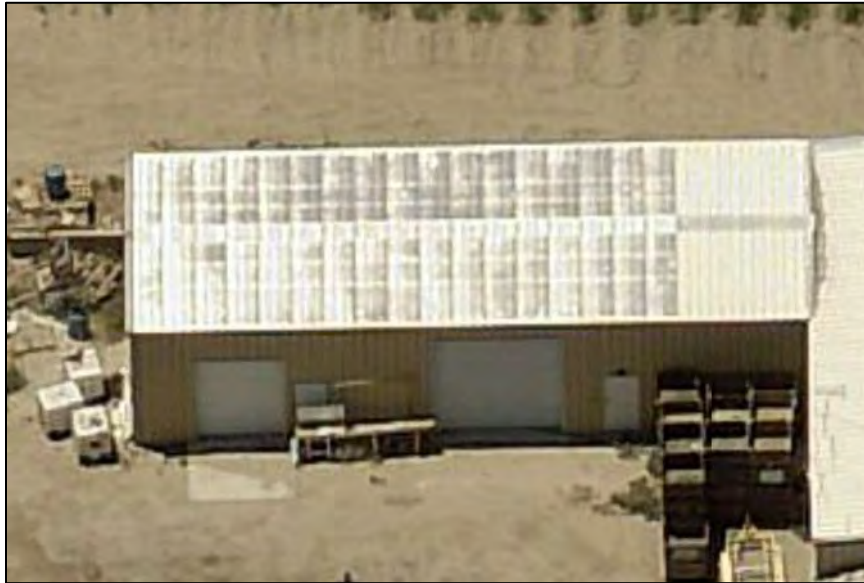
Photograph 27: Aerial view of the east side of Building H (EagleView Technology Corporation 2020).
