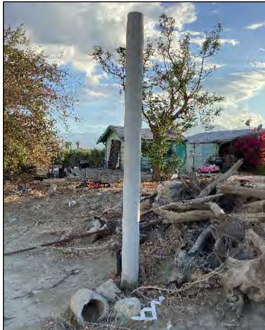
Photograph 5: Exposed concrete pipe located northeast of the residence (Building A). Camera facing southwest, October 6, 2022.
