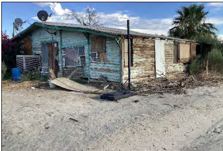
Photograph 9: North and west sides of Building A, showing a mix of original and replacement window fenestration. Camera facing southeast, October 6, 2022.
