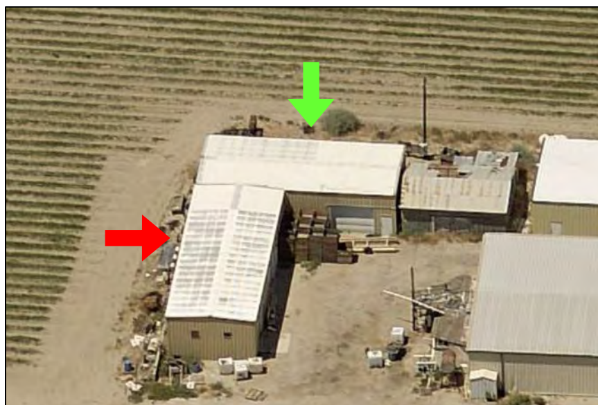
Photograph 26: Aerial view of the south sides of Building G, marked by the green arrow, and Building H, marked by the red arrow (EagleView Technology Corporation 2020).
