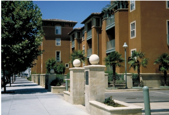
Three-story apartment complex with a landscaped setback.
